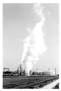
several wells were drilled to depths of 5,000 to 8,000 feet. In the Salton Sea geothermal field, typical brines are produced at wellhead temperatures up to 600°F. During extraction, the high temperatures and reduced pressure in the drill holes cause the superheated water to flash into steam, thus bringing in a mixture of steam and hot water at the wellhead.
