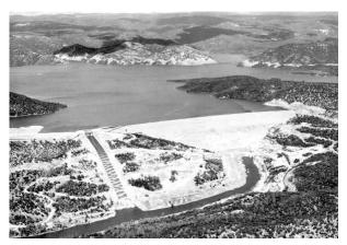
picking up pollutants and salts. Many of the facilities in the state water system are unprecedented in size. There is the Oroville Dam, more than a mile wide at its crest and 747 feet high. The dam, with its spillway is the highest earthfill dam in the world. The leading structure in the system, however, is the California Aqueduct, 444 miles in length. The physical plant of the total planned project is about 60 percent complete. The principal requirements not yet constructed are additional major
