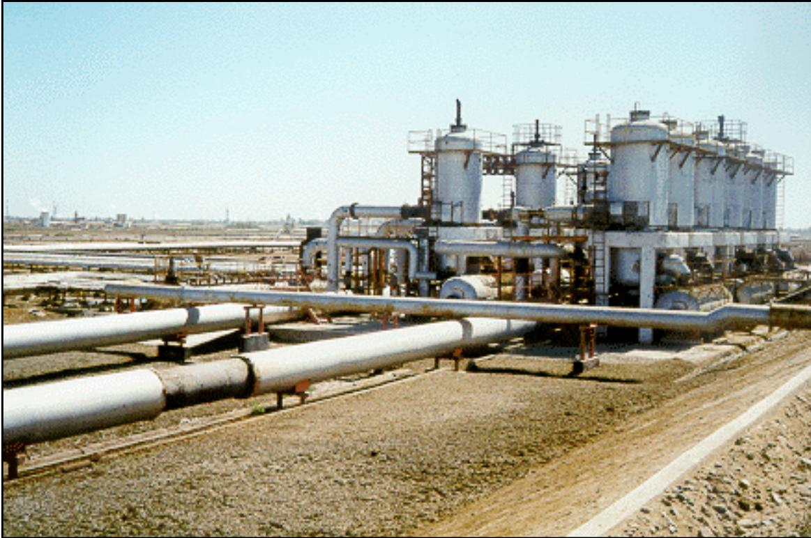
The Cerro Prieto geothermal field generates 620 Megawatts of electric power and in the process pumps 2.6 million gallons (U.S.) (11,000 metric tons) of brine water from underground per hour that is disposed of in surface ponds. Evaporation removes most of the water quickly leaving approximately 1300 metric tons of silica waste as the residual product from this hourly production of brine. At present, there is no use for this waste silica.
