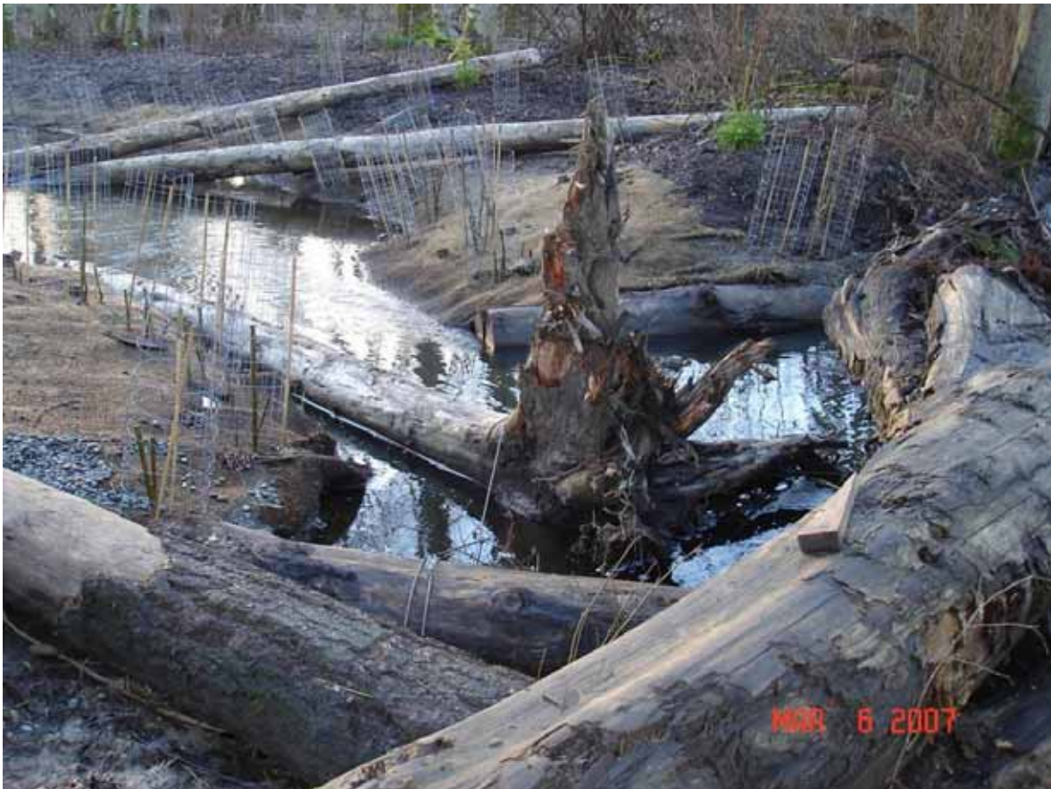
Figure 2-1. Photo showing recently constructed stream channel in Cemetery Creek, with newly planted conifers, willow stakes and deciduous shrubs; March 6, 2007.
